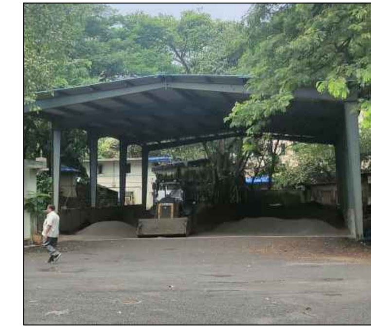
IMAGE REFERENCE: ADJACENT SHED TO NEW OFFICE
