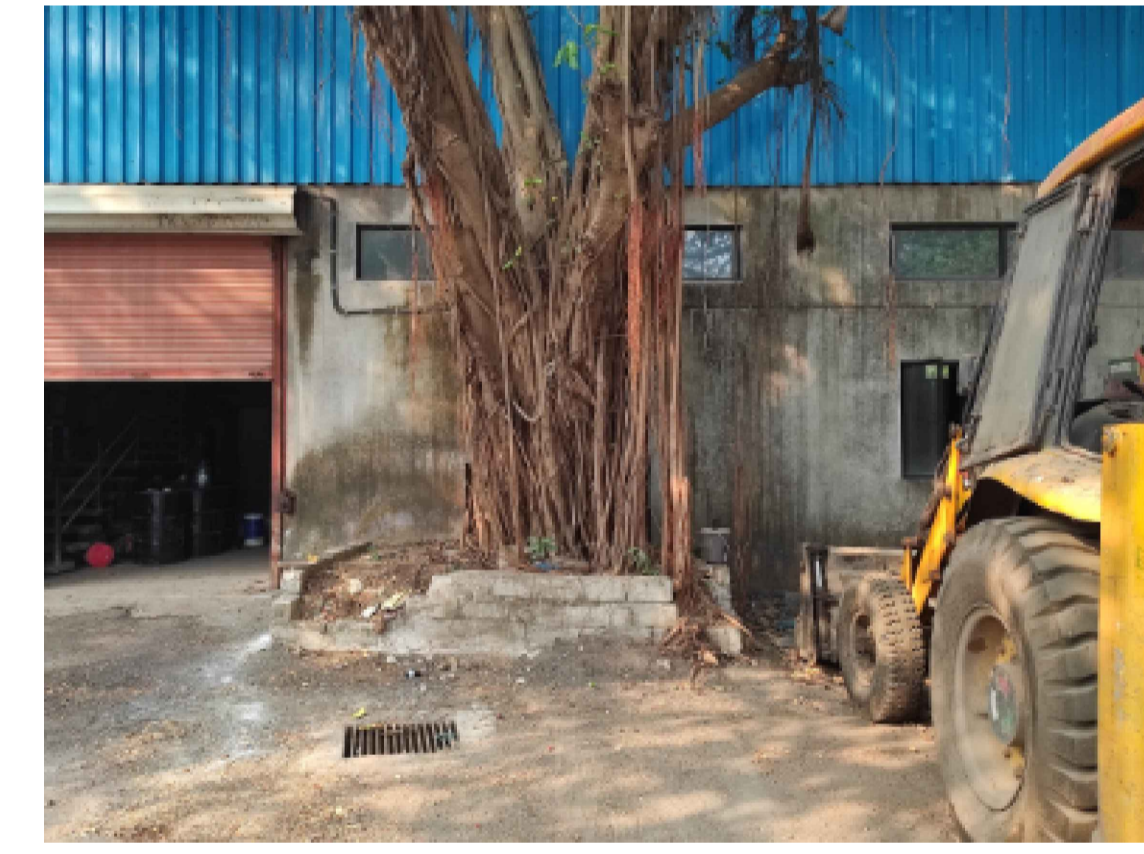
IMAGE REFERENCE: ROLLING SHUTTER 1: PROPOSED ENTRANCE TO CONCRETE SECTION
