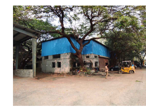
IMAGE REFERENCE: NEW OFFICE BESIDE SHED
